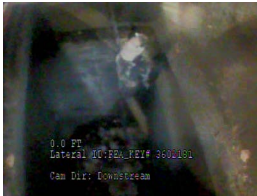
Auger in the outfall
