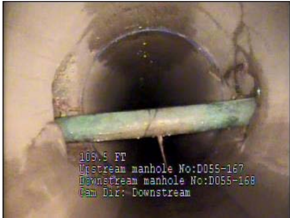
Water service meets drainage pipe
